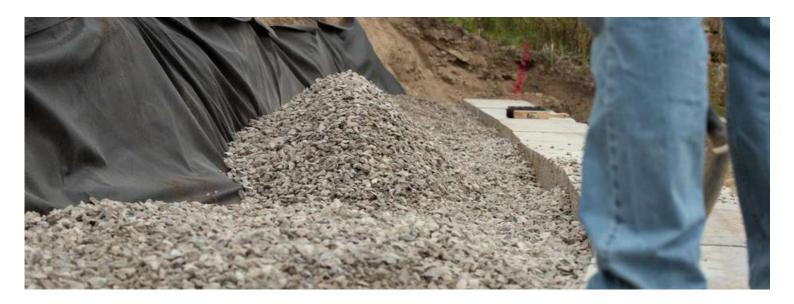
Appropriate selection and placement of backfill is necessary for the structural integrity of the wall. **Place only backfill materials which are consistent with the wall design.** For safety reasons, do not stack wall blocks more than 3 feet (0.9 meters) high before backfilling. <u>See Figure 2.</u>
